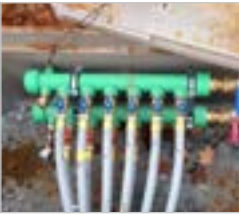
M-8400 GeoGreen™ mounted ground vault
