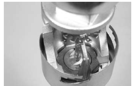
CORRECT ENGAGEMENT FOR MODEL V36 CONCEALED/RECESSED WRENCH
